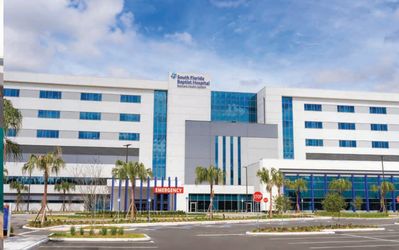
The replacement hospital for South Florida Baptist Hospital, located four miles from the original hospital, will open in east Hillsborough County in the second quarter of 2024.
